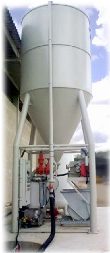
Water Treatment Plants by F&B Separates the waste product & water; recycled water returns for use. Systems eliminate sludge pits/monthly cleaning.
